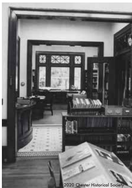
Library 1961 view across 1st floor
